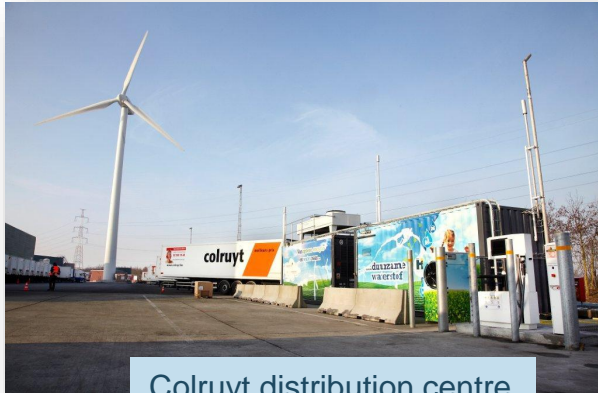
Colruyt distribution centre From wind-solar
